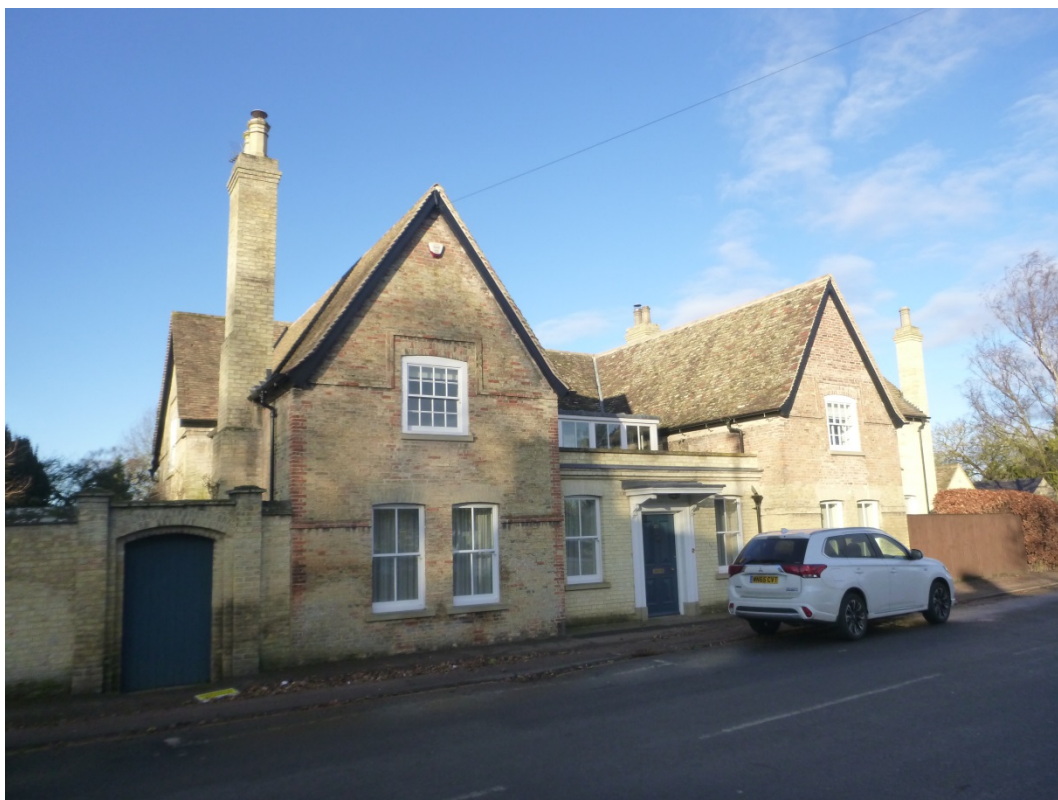
Photograph 7 - The above photograph demonstrates the architectural role of listed buildings along High Street at Waterbeach.
